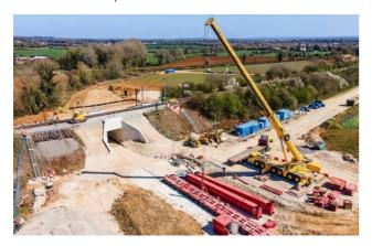
During a 100-hour railway closure between 2 and 5 April, the railway embankment was removed and two prefabricated structures - a steel underbridge and a concrete underpass with a combined weight of 2,200 tonnes - were inserted using remotecontrolled transport.
